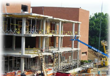
Fig. 1 - 6/7/07: Curtainwall and storefront installation on east elevation
