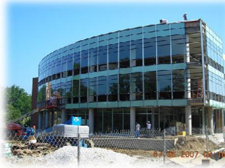
Fig. 5 - 7/6/07: Glass installation on south elevation, excluding fritted glass
