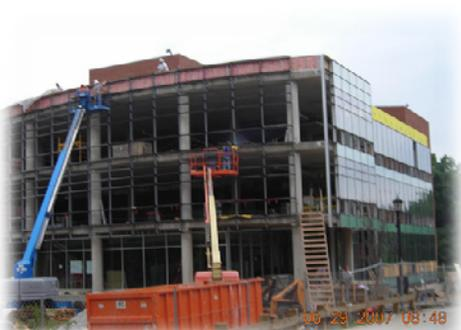
Fig. 4 - 6/29/07: Curtainwall grid installation on south elevation
